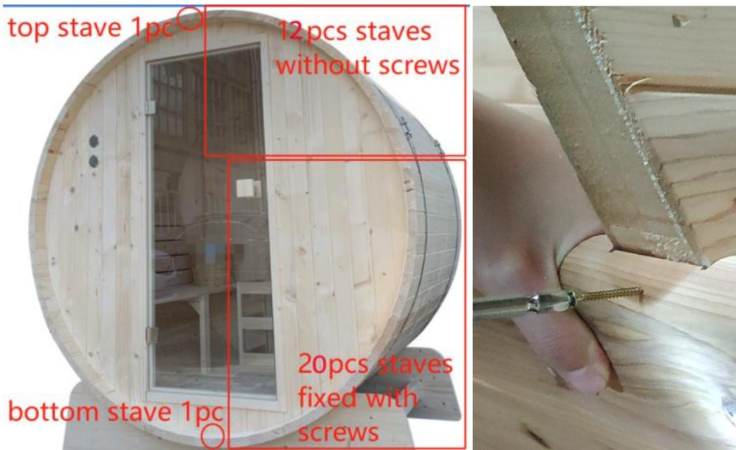
9. Top piece provided with 2 sizes. Choose the one that fits. After the top piece is well installed, fix all the staves with screws.
