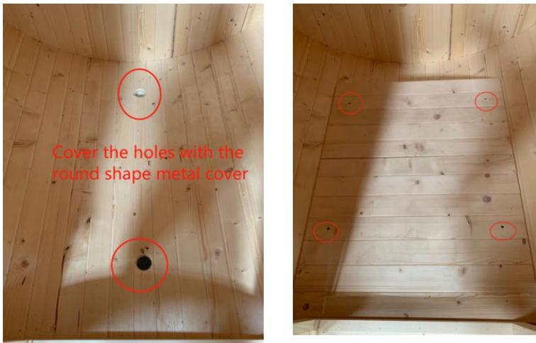
12. Install the seat with 4\*40mm screws.
