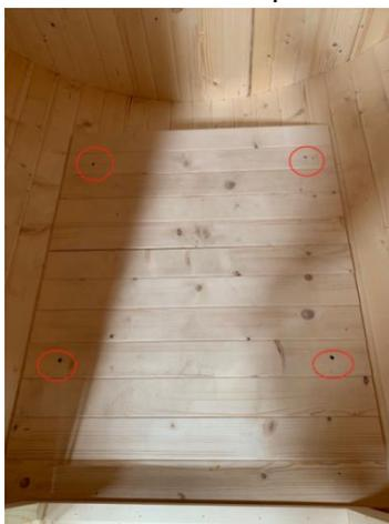
12. Install the seat with 4\*40mm screws.
