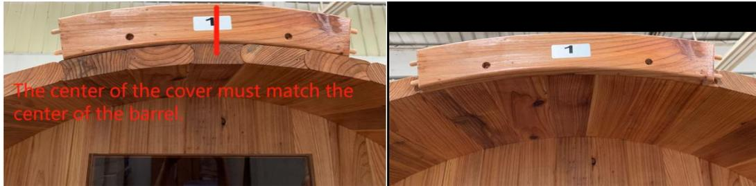
The center of the cover must match the center of the barrel.
